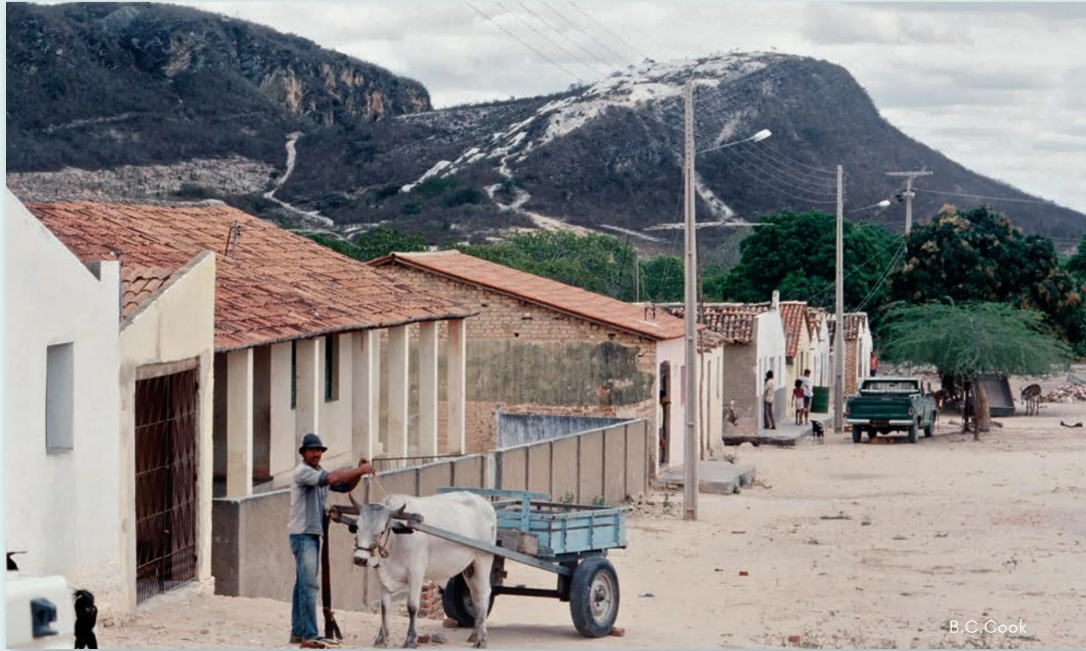
From the village of São José da Batalha, one can see the original mine with its white kaolin clay tailings piles on top of the granite massif.
